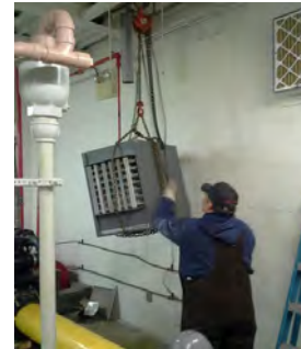
Airport pump station heater replacement
