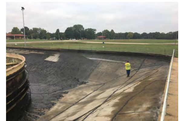
Basin Cleaning Completed
