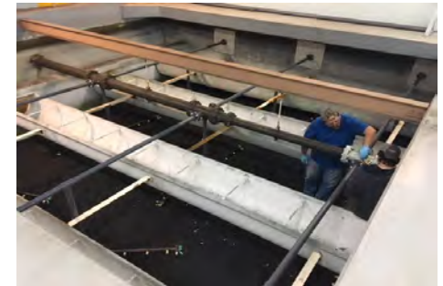
Replaced surface wash lines on #2 and #3 filter
