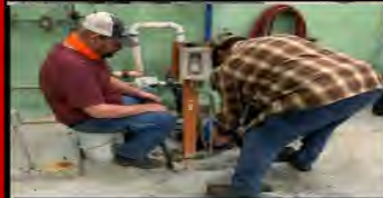
Installed New Seals In Carbon Pump
