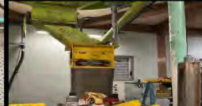
Rebuilt Lime Feeder
