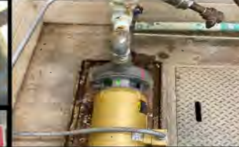
Installed New Screen Wash Pump
