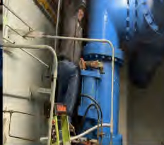
Started Dismantling #2 Backwash Pump for Rebuild
