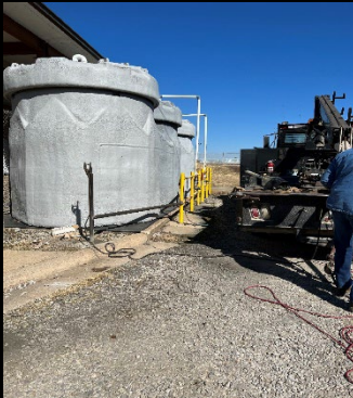
Extended the railing Around the Alum Storage tanks.
