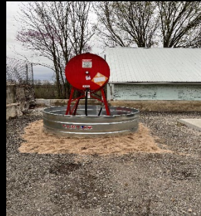
Set fuel tank into containment tank.
