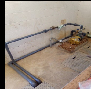
Installed new suction And discharge lines to the screen wash pump.
