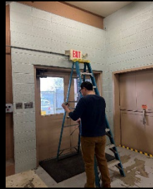
Checked batteries on all emergency exit lighting.
